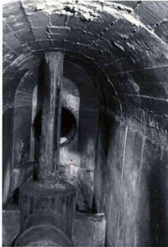
Figure 41: Photograph of Bulkhead No. 1 (STA 0+30) - From Bowles Planning Report
