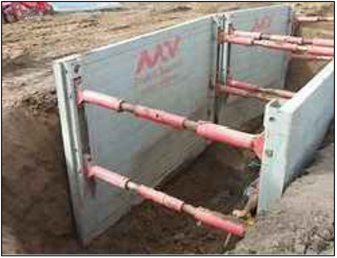
TYPICAL TRENCH SHIELDS NOT TO SCALE
