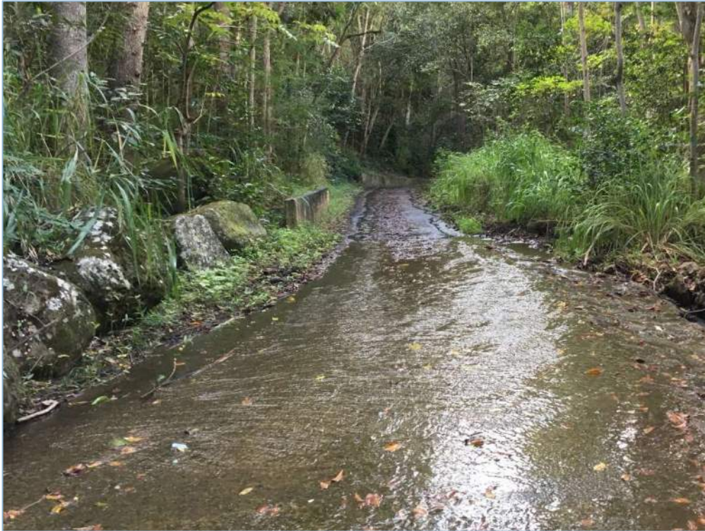
Figure 1-6. Water flowing over Access Road due to Blocked Pipe Culverts (photo provided by Bills Engineering)
