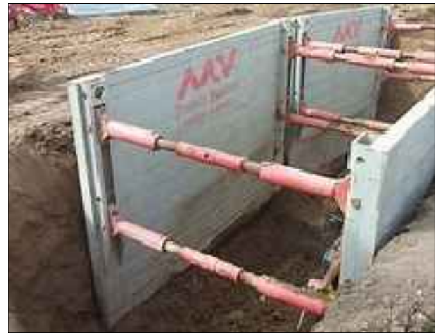
TYPICAL TRENCH SHIELDS NOT TO SCALE
