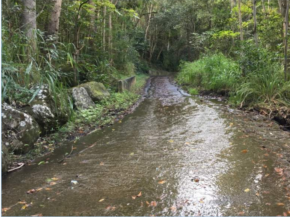
EXHIBIT 6 WATER FLOWING OVER ACCESS ROAD DUE TO BLOCKED PIPES
