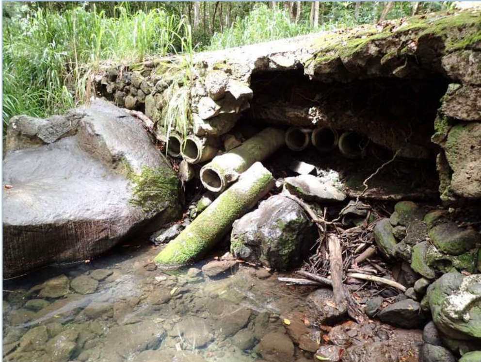
Figure 1-2. Makai Side of Access Road showing Erosion Damage
