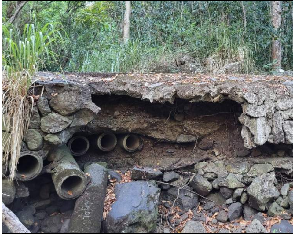
Figure 2. Downstream scour exposing small diameter pipe culverts beneath Ford No. 2
