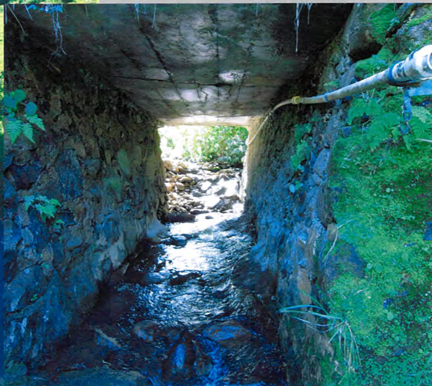
Existing Unlined Culvert (Looking from Downstream End)
