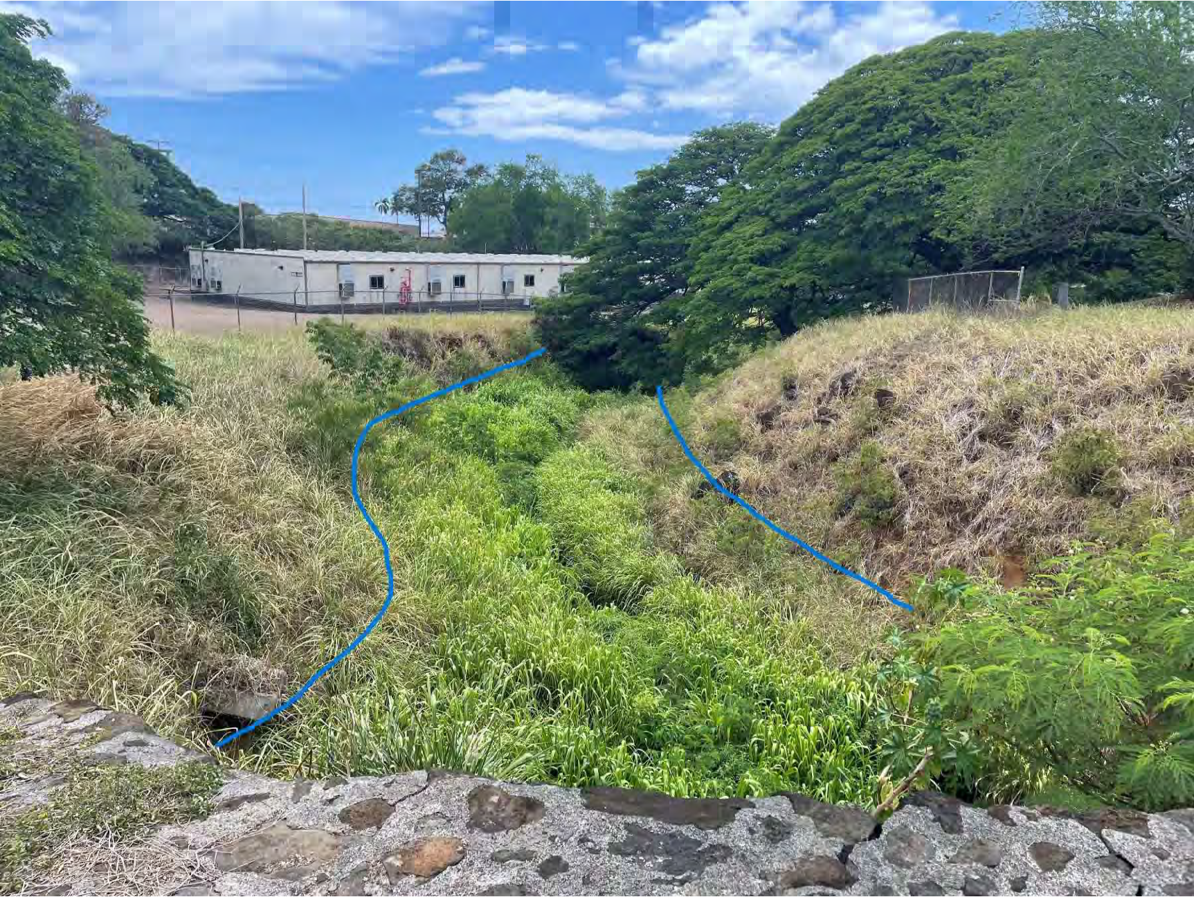
Photo 2 - Kahauiki Stream with OHWM facing SE from Morton Drive Culvert
