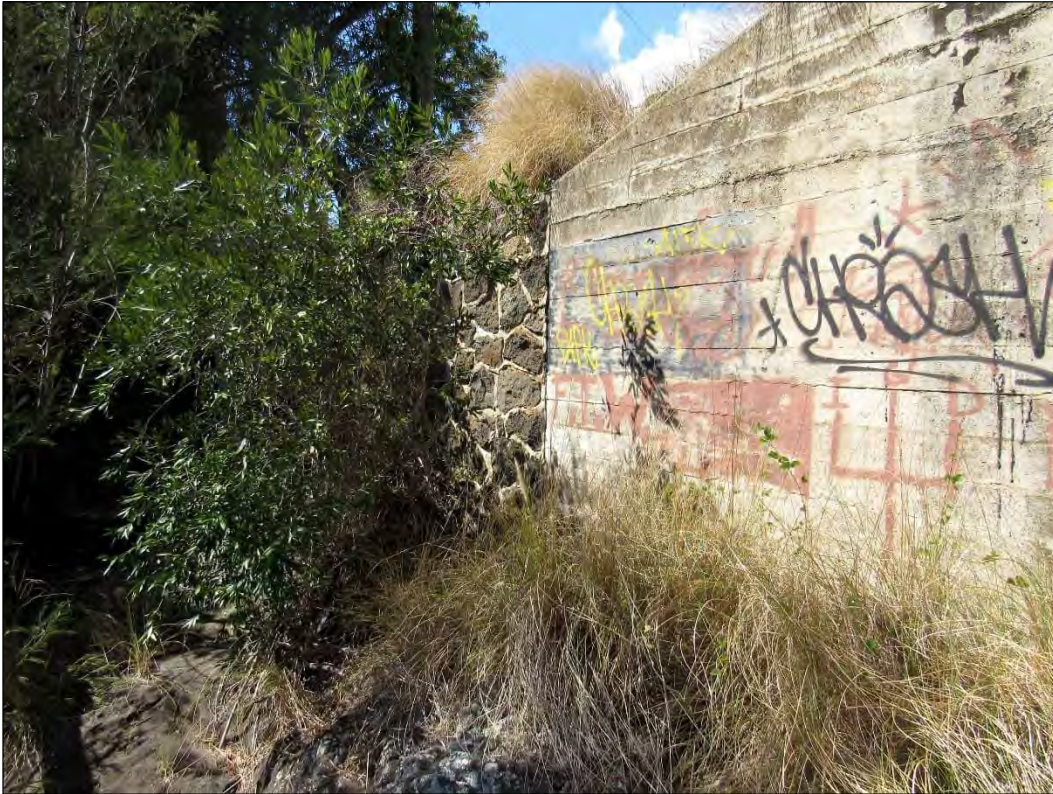
Figure 34. SIHP 50-10-06-29221 Wai'aka Bridge concrete and masonry abutment wing walls, view to the northwest.
