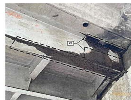
6 PHOTO - GIRDER CORROSION AT WAILUKU ABUTMENT NOT TO SCALE
