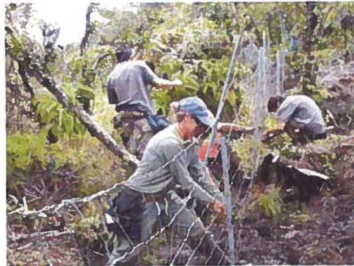
Installing fence in East Maui's watershed
