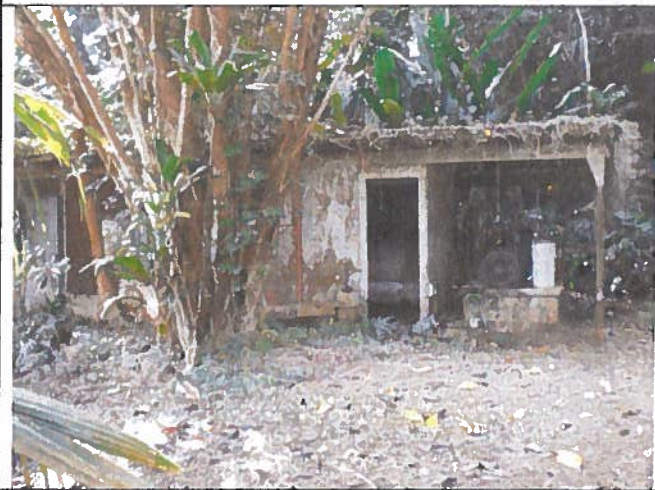
View of shed situated mauka of dwelling.
