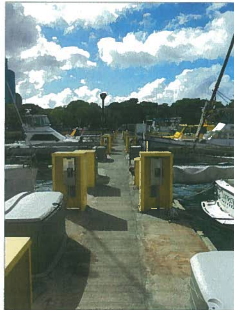
4 Pier A looking east.
