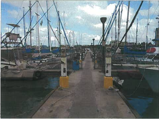
5 Pier B looking west.
