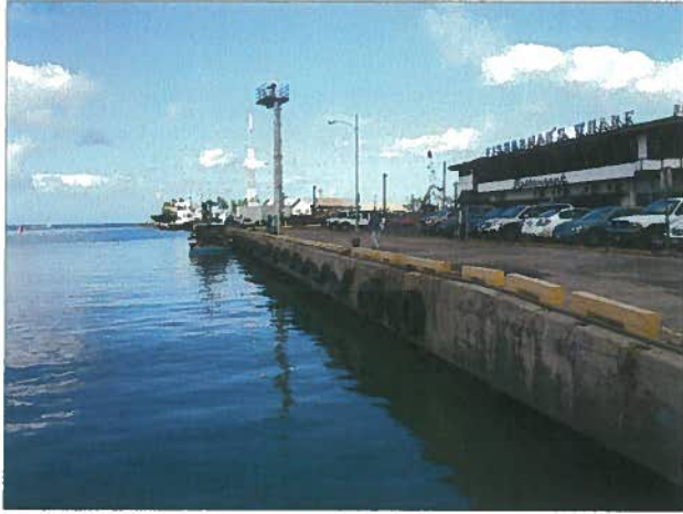
1 'Ewa Loading Dock and former Fisherman's Wharf restaurant.
