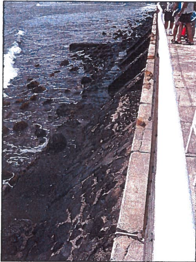
Photograph No. 3: Revetment footings of swimming pool (Easement "E-3")
