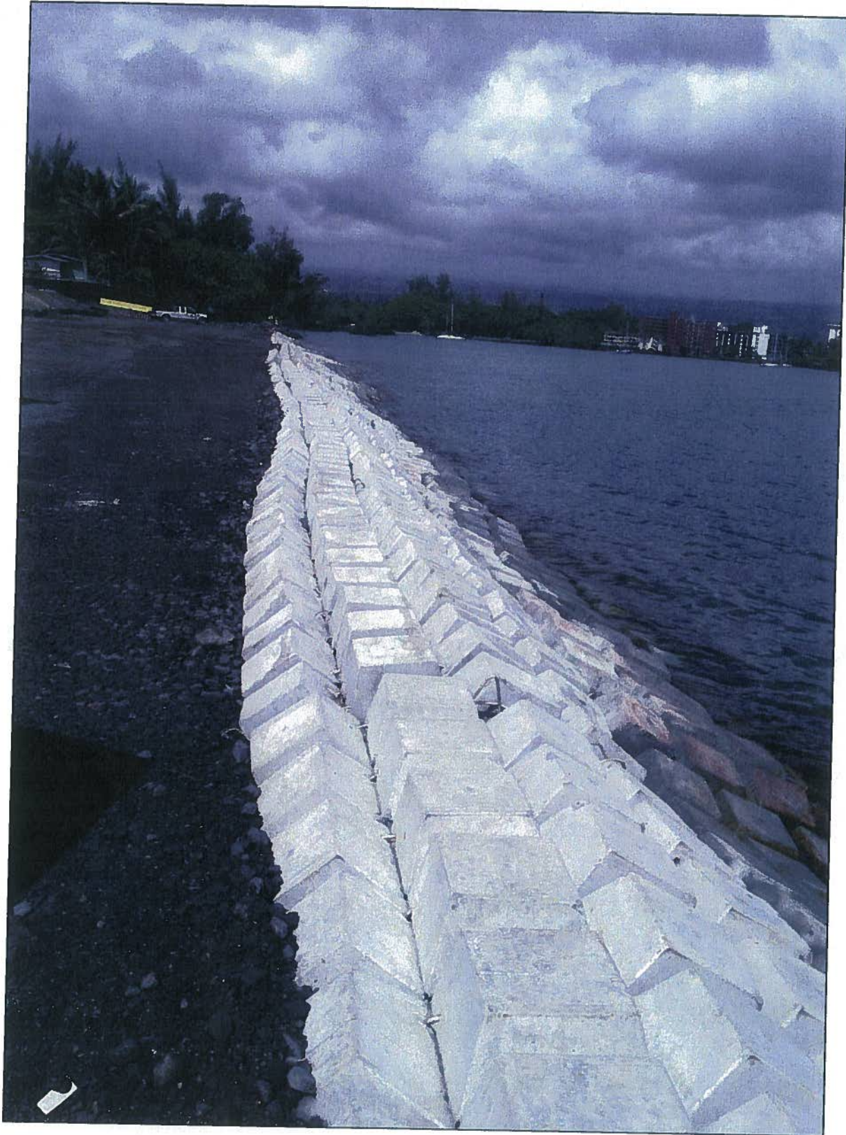
Views of the shoreline where Pier 4 would be constructed.
