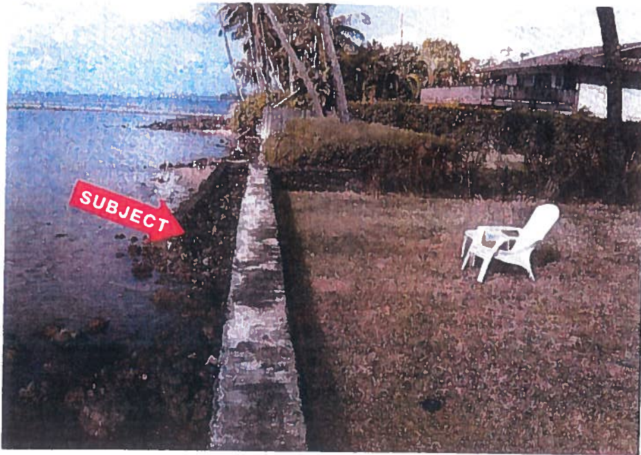
PHOTO NO. 5: Westerly view along the southern boundary of the Reclaimed Land. Note that the rock outcropping at the base of the wall is included in the Reclaimed Land.
