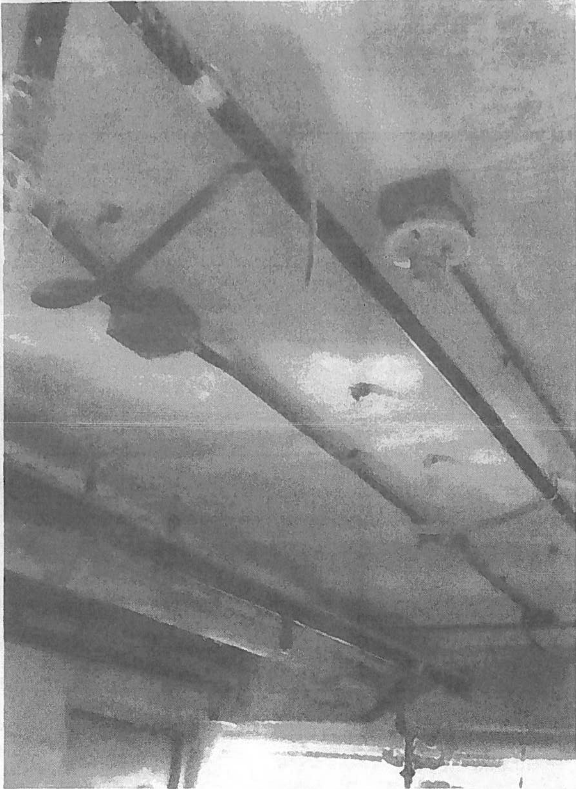
Exhibit U - ART 372.13 Discontinued outlets. Circuit conductors shall be removed from the raceway, Art 410.3 Live Parts. Luminaires shall have no live parts normally exposed to contact
