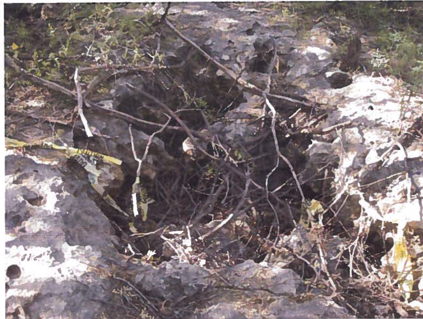
Figure 3: Sinkhole filled with debris
