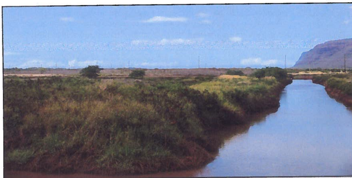
Main drainage canal at Kawai'ele pump station.
