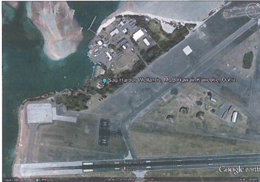
Figure 3.10 - 3. Sag Harbor Wetland at Marine Corps Base Hawai'i at Kaneohe on the island of O'ahu in relation to runway 04/22.
