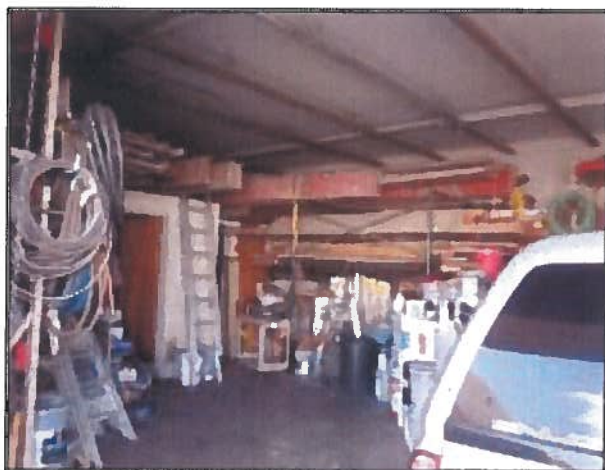
INTERIOR VIEW OF UNIT 104
