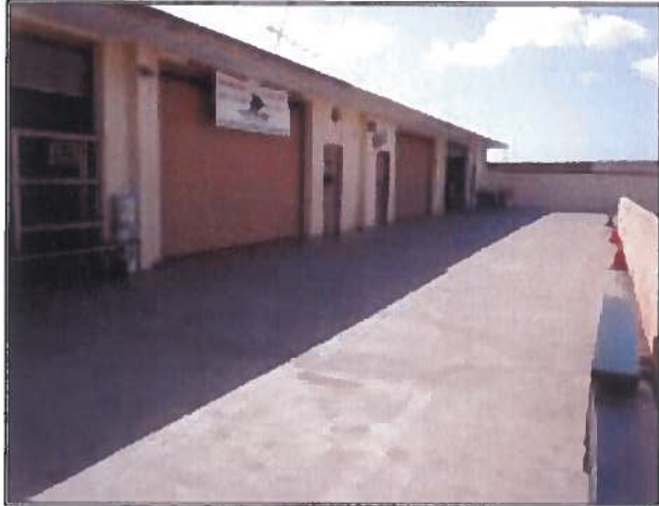
ANOTHER VIEW OF 2 ND FLOOR
