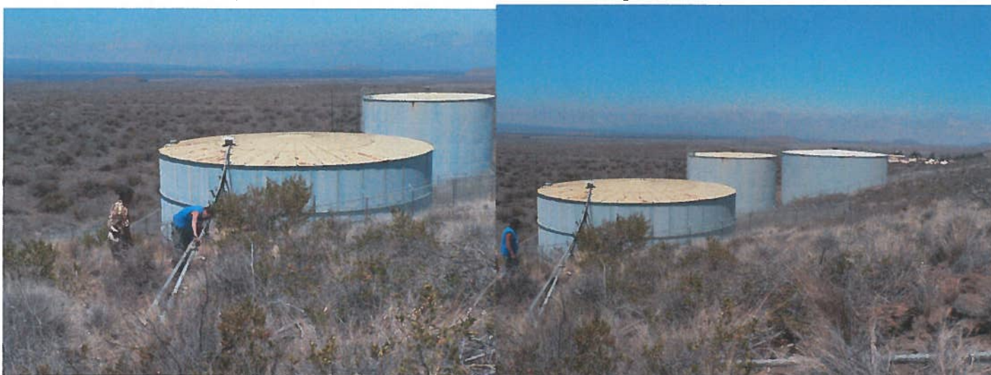
Photos of main feed storage tank and overflow tanks connected in sequence
