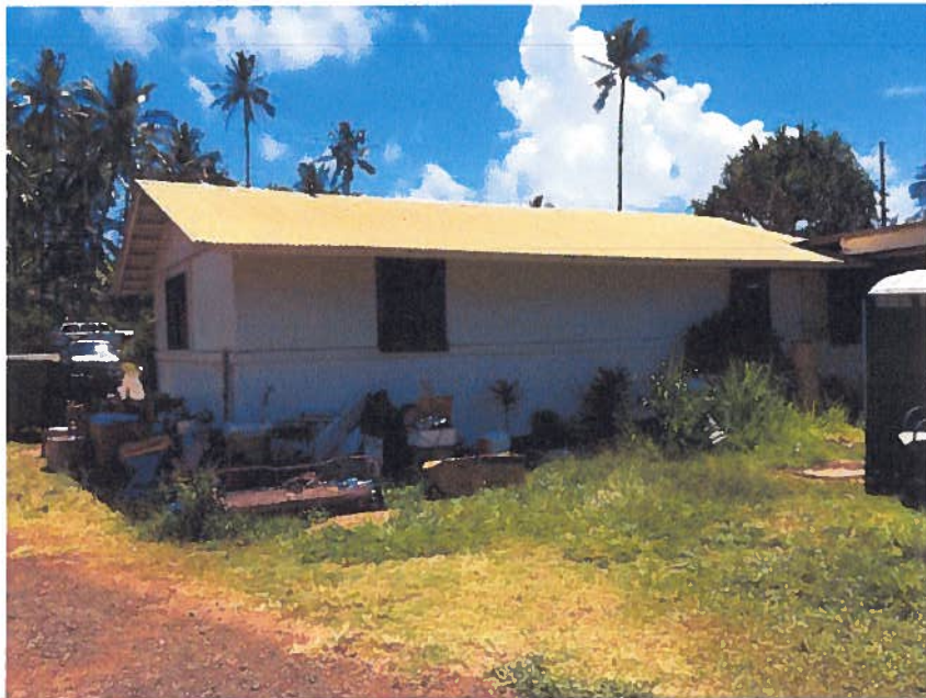
Elevation facing northeast
