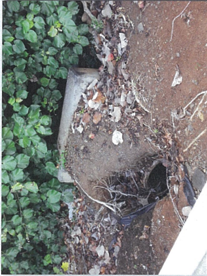
Photo 2: Northeast view of Culvert 1 condition.
