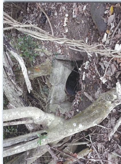
Photo 6: East view of Culvert 3 condition.
