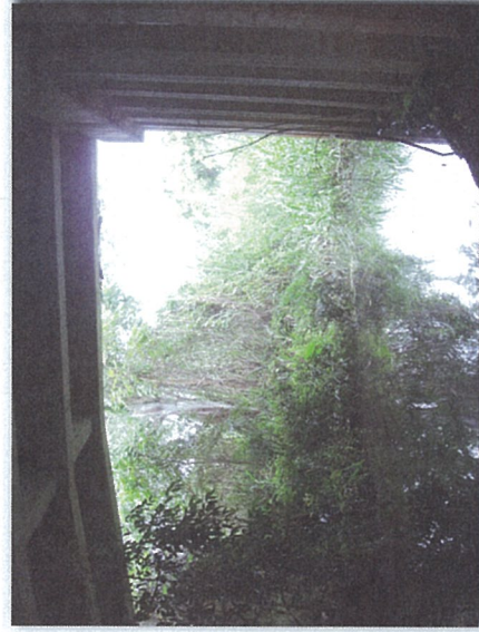
Photo 4: South view of Kahanaiki Stream under highway bridge.
