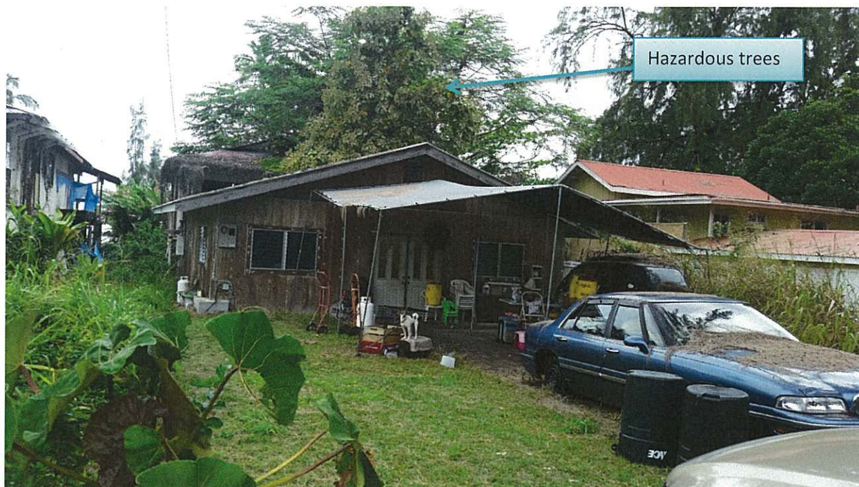
View from street – note overgrown trees on roof. Two inoperable vehicles sitting in front yard area.
