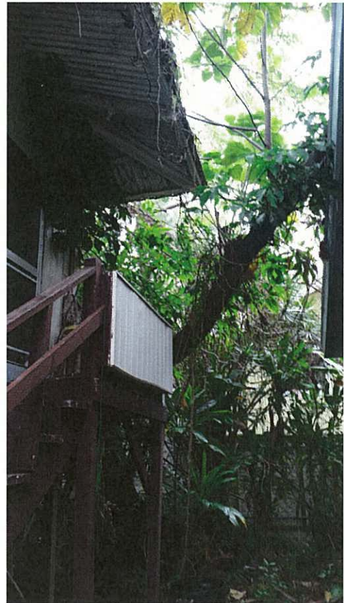
Entry stairs to original house – note trees and vines on both structures.
