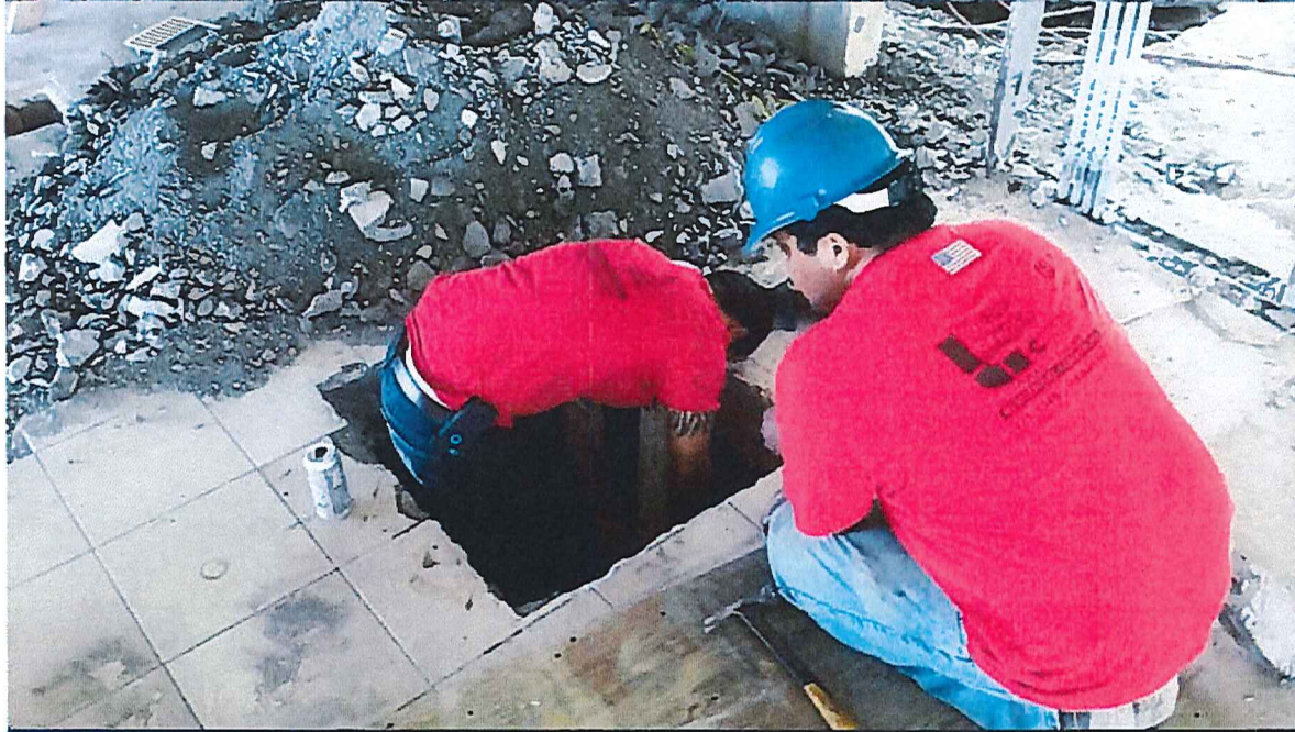
Water feature demo and waste line repairs
