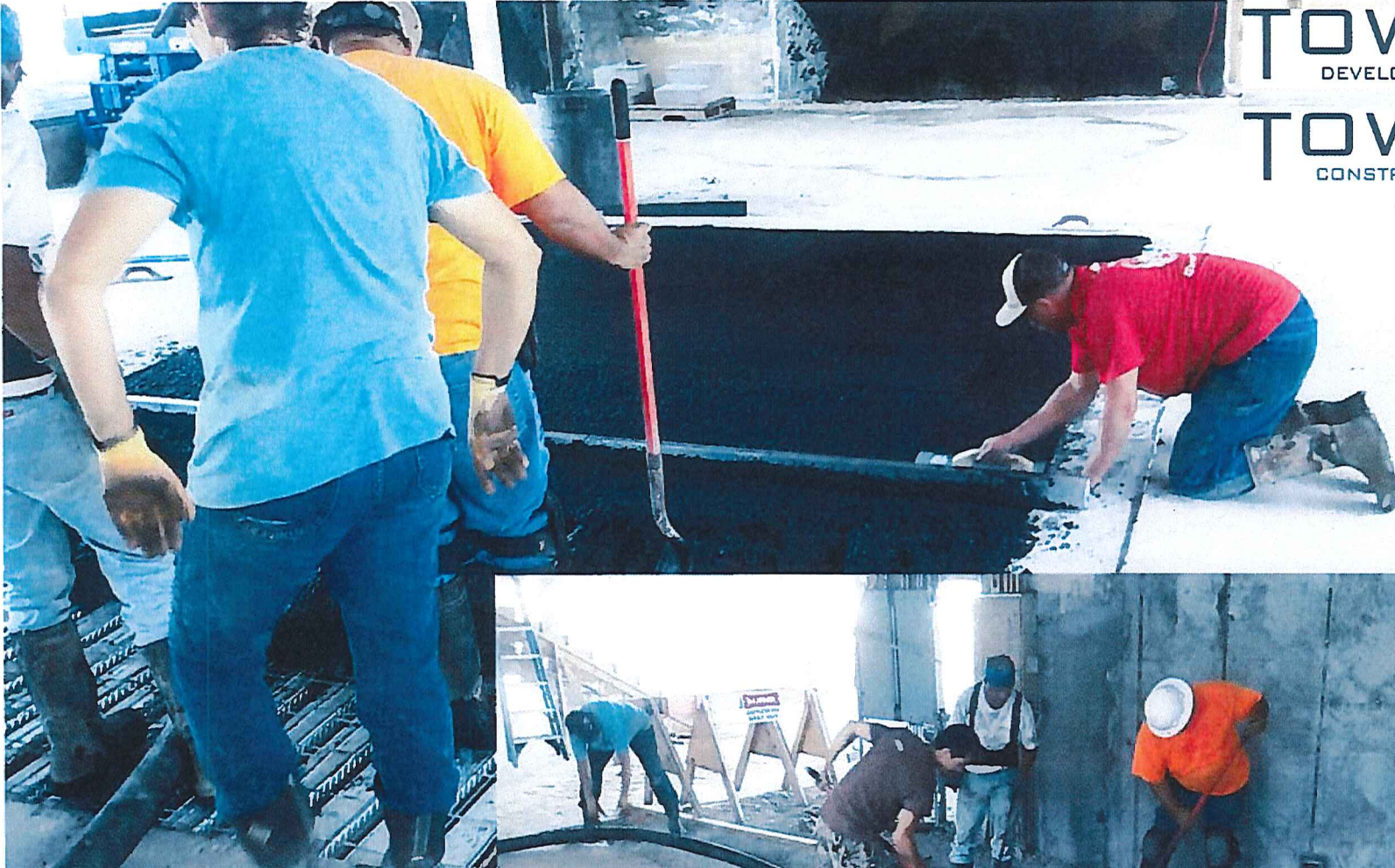
Upper and lower level slabs placement
