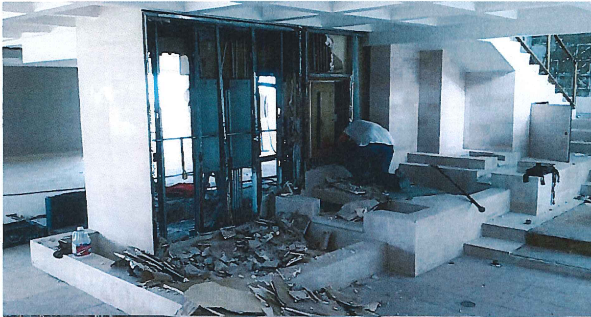
Lower wall, stair, and water feature demolition
