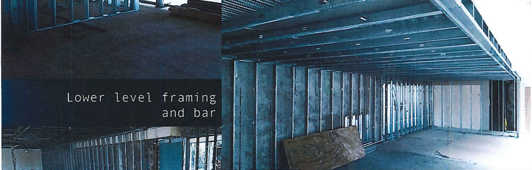
Lower level game room wall and ceiling framing and preparation for sprinkler installation
