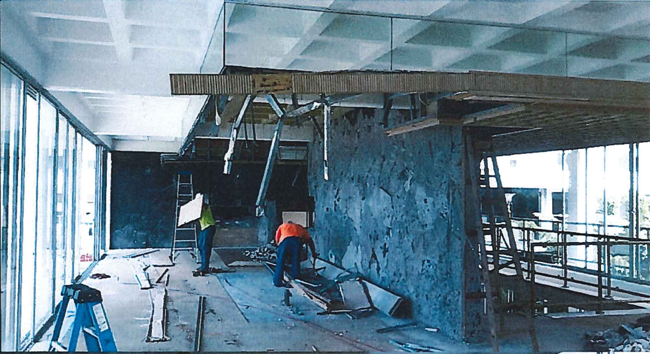
Center concrete wall demolition
