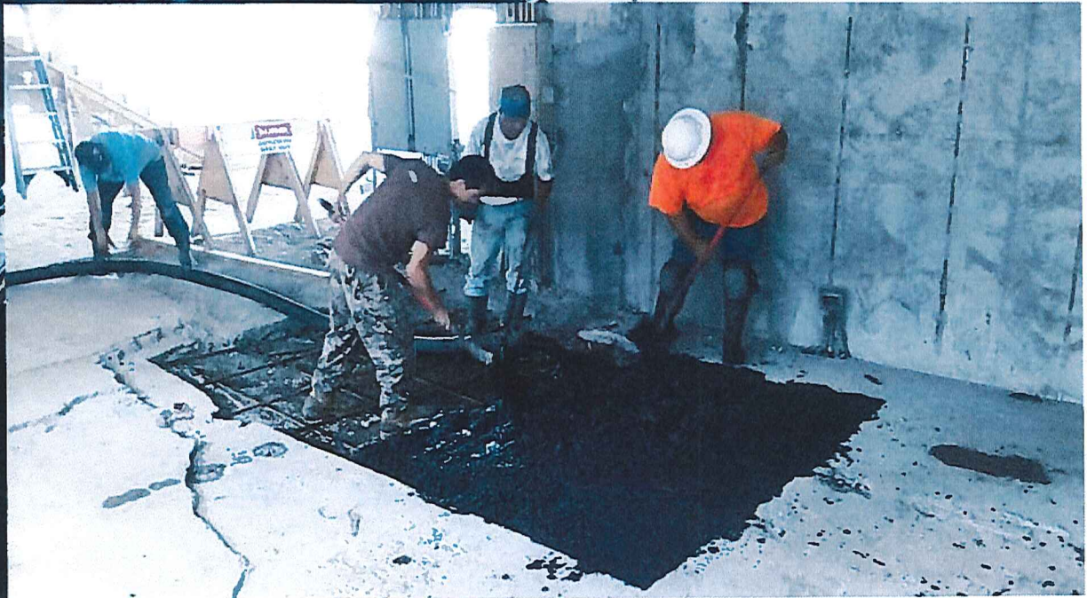
Upper and lower level slabs placement
