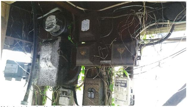
Main electrical panel and breaker box mounted under original house.
