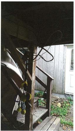
Electrical wiring and switches hanging under original house.
