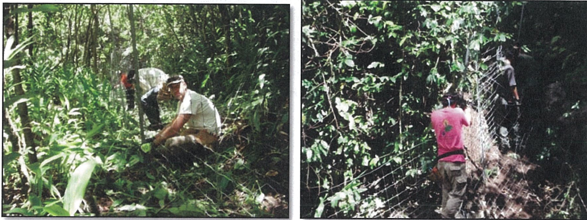
Figure 6. New Honokōwai Valley fence installed in FY14.
