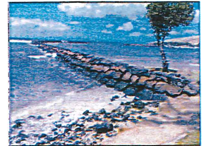
Photo of Ma'alaea breakwall.
