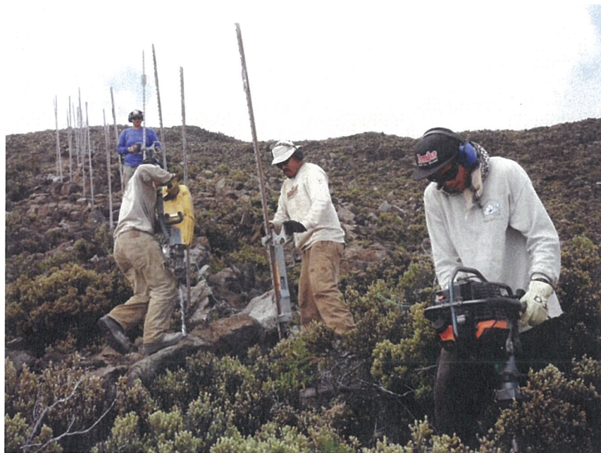
Figure 17. Installation of fence unit in upper Nakula NAR.
