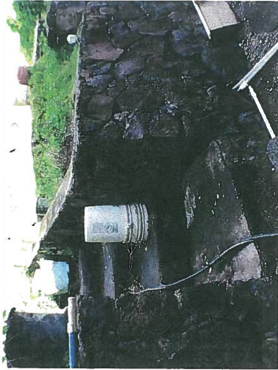
Retaining wall requested to remain; Steps & side walls to be removed; New retaining wall to fill opening
