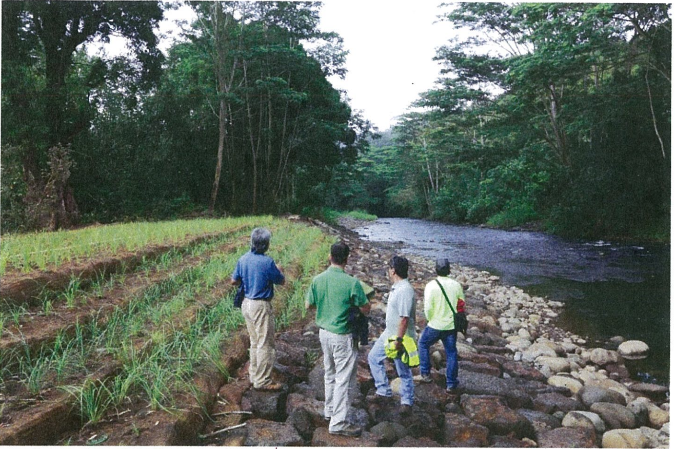
Breach Repair Project – Final Inspection
