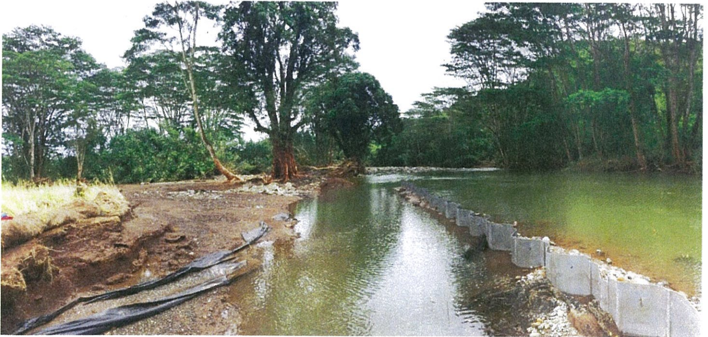
Breach Repair Project Site – After April 2018 Flooding
