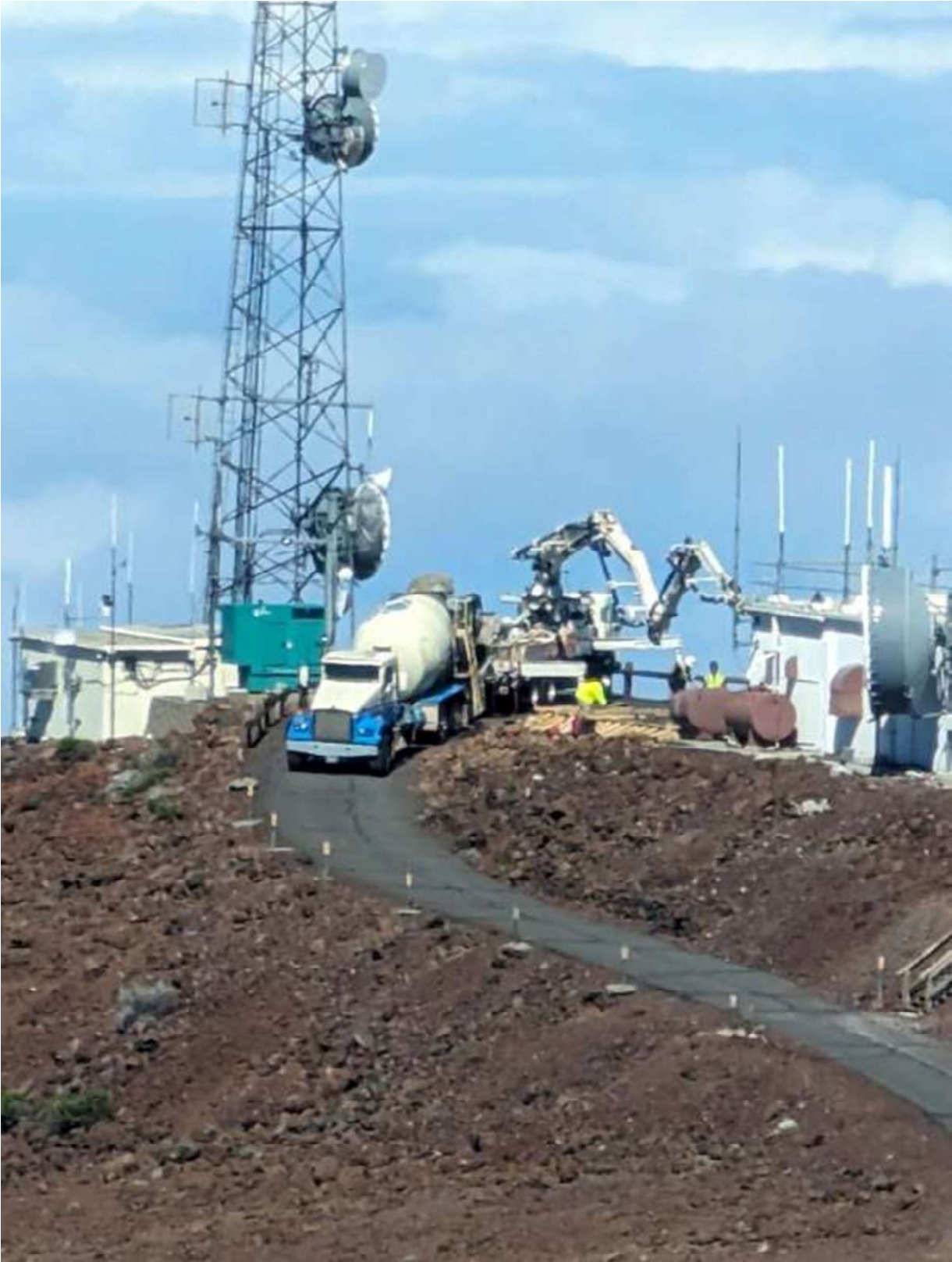
FAA Antenna Site Under Repair, SPA MA-20-63, TMK (2) 2-2-007:007, EO 1413
