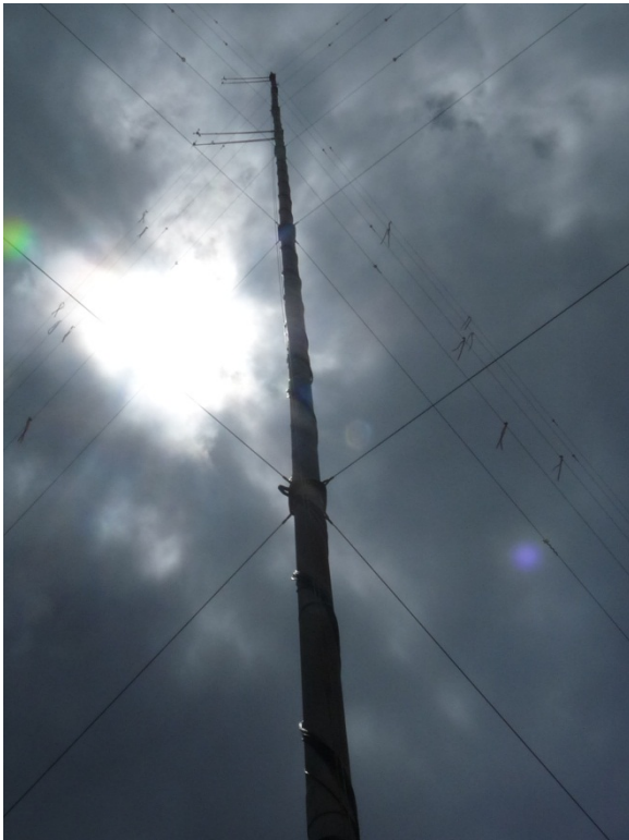
Figure 8. Guy wires on one of the meteorological towers on Lānaʻi, covered under the HCP. Guyed towers pose a much higher collision risk for seabirds and bats than do unguyed towers.
