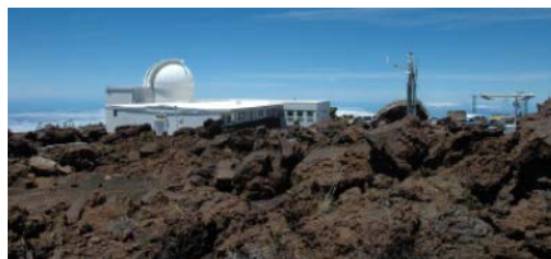
ATST construction site. Maui, Hawai‘i.
