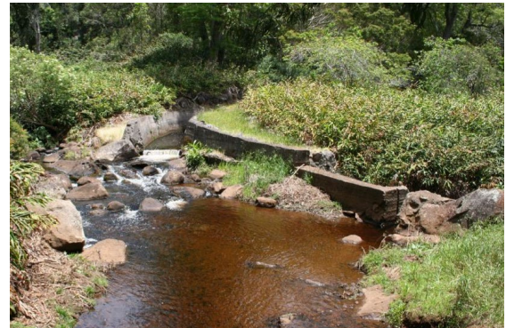
D) Diversion dam at Kōke'e Stream.
