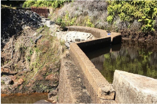
A) Diversion dam at Waiakoali Stream.
