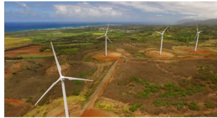
Kahuku facility on the North Shore of O'ahu.
