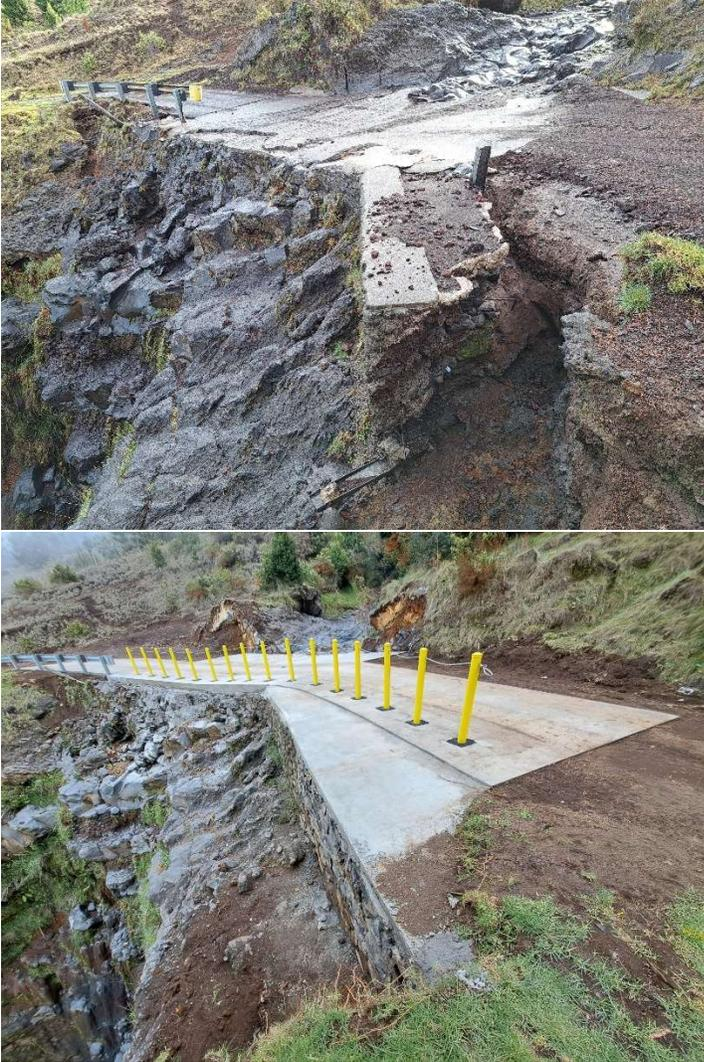
Figure 3. Storm damage to a cement stream crossing on Waipoli Road in the KFR and the same crossing after repairs.
