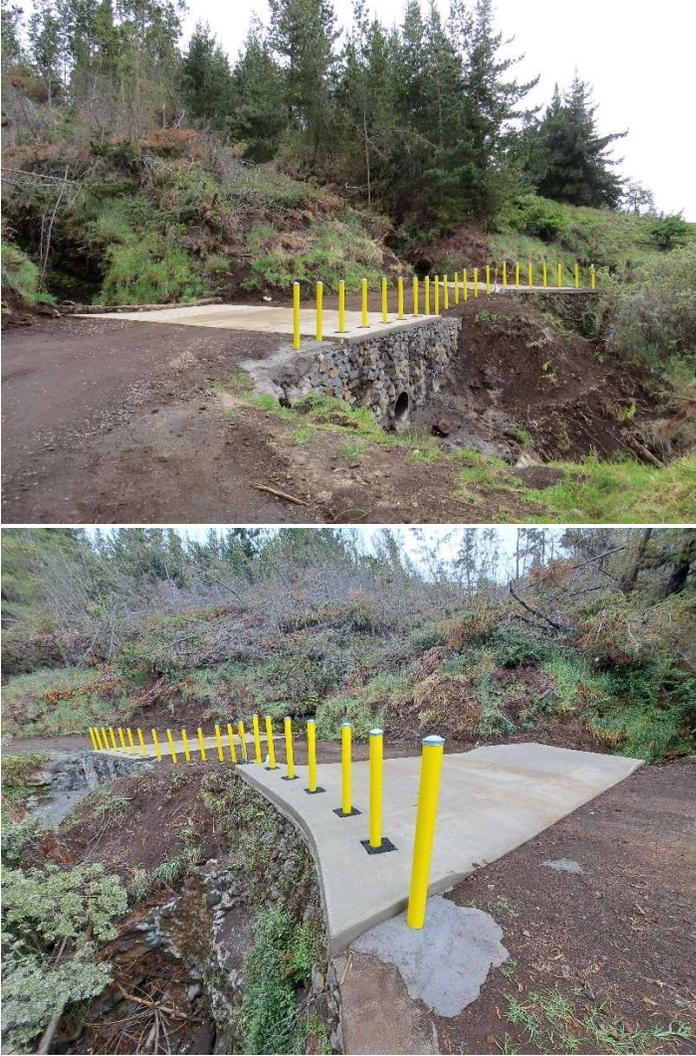
Figure 4. Newly reconstructed culverts and spillways after repairs.
