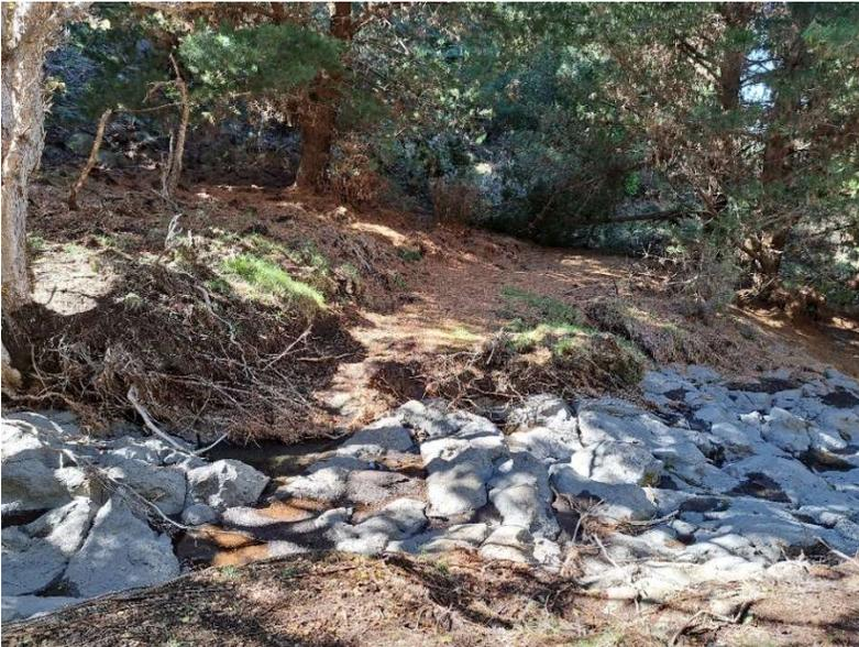
Figure 5. Kona Low Storm damage to stream crossing spillway #6.
