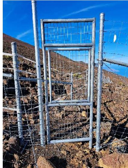
Figure 8. Kamehamenui Forest Reserve fencing and pedestrian walk-through gate.
