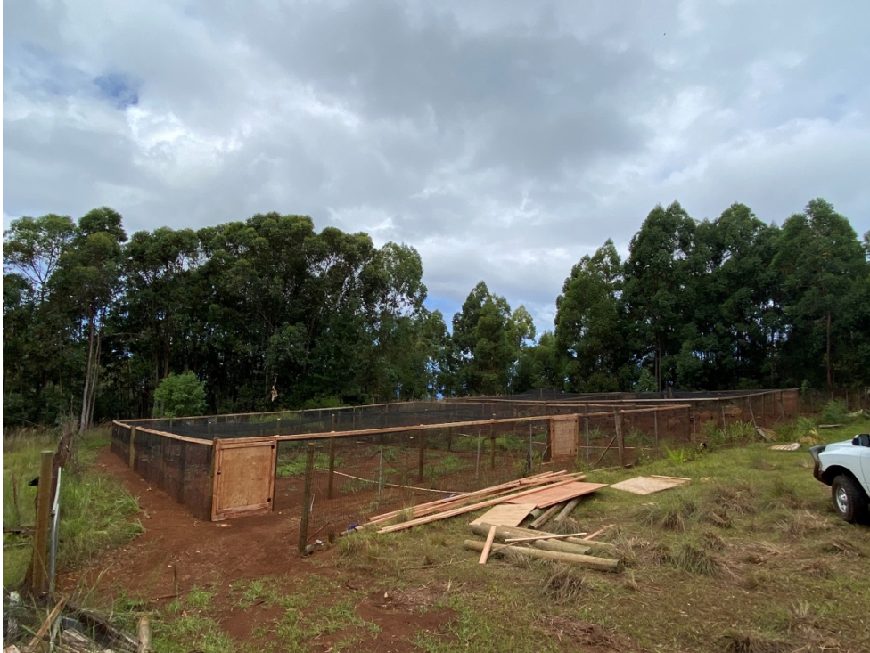
New fly pens constructed, Kauai
