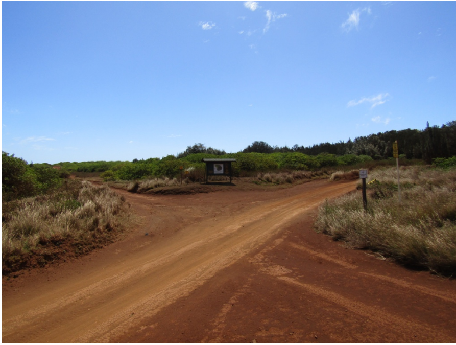
Roads maintained on Lānaʻi
