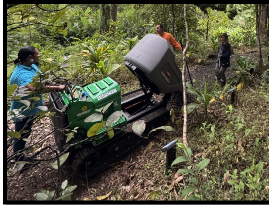
FIGURE 6: NAH STAFF HARDENING THE TRAIL BY LAYING GRAVEL WITH A MECHANICAL WHEELBARROW
