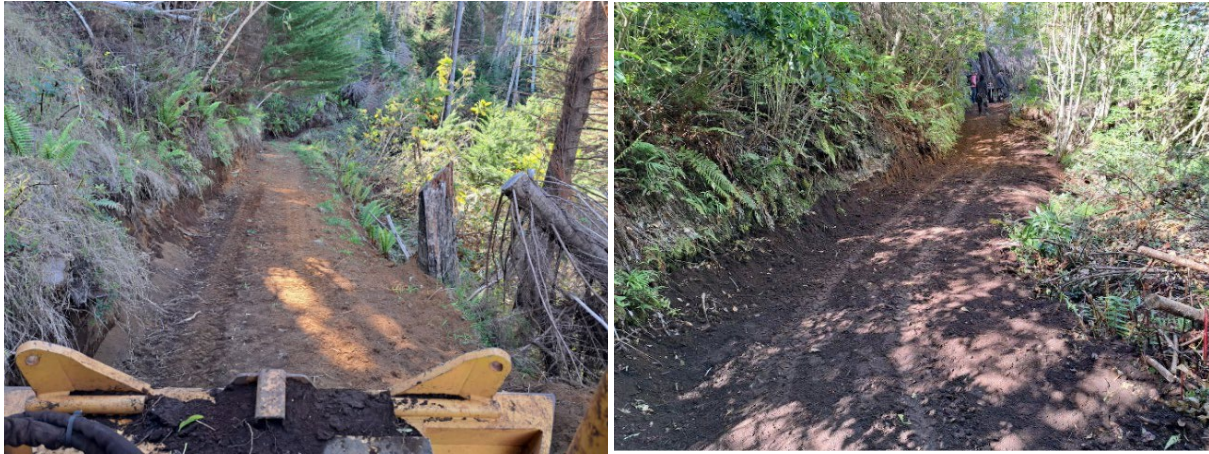
Trail dozer tread work on Plum Trail in KFR.
