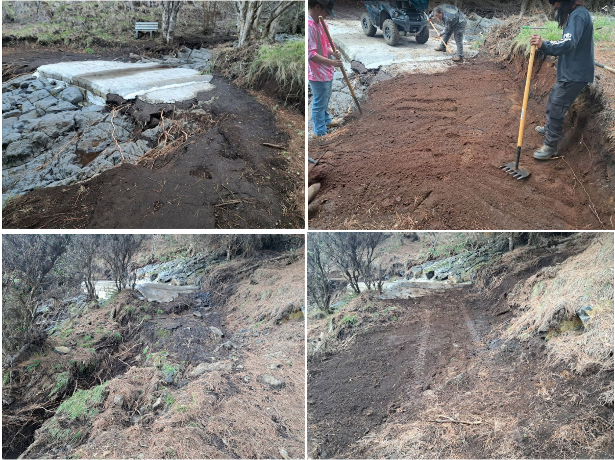
Waiakoa Loop Trail tread repair before and after.
