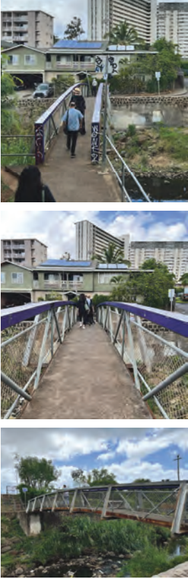
EXISTING BRIDGE AT RICHARD LANE:
