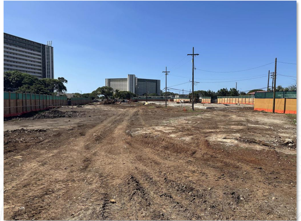
All existing buildings have been completely demolished
