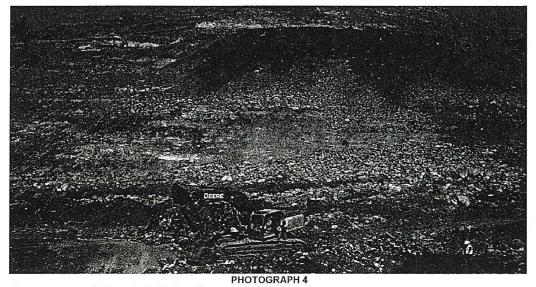
Site name: Location: Date taken: Photographer: Description: Waimanalo Gulch Landfill 94-460 Farrington Highway January 24, 2011 JRuiz On-going construction of the upper Cell E-6 (blue arrow) has added to the damage sustained by the western portion of Cell E-6 liner (red arrow).
