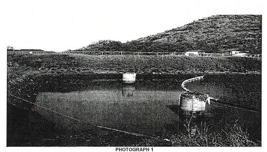
Waimanalo Gulch Landfill 94-460 Farrington Highway February 1, 2011 JRuiz Sedimentation basin with 7 ½ feet of liquid still remaining. WMH continues to pump and transport the liquid to Waianae WWTP.
