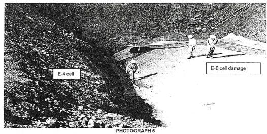
Waimanalo Gulch Landfill 94-460 Farrington Highway January 24, 2011 JRuiz Contractor working on damaged Cell E-6 liner.
