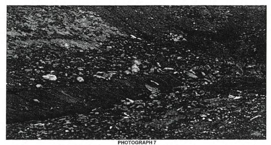
Waimanalo Gulch Landfill 92-460 Farrington Highway January 18, 2011 JRuiz Closed-up view of the damaged liner to MSW Cell E-6 due to the rainstorm and earlier upper cell construction.
