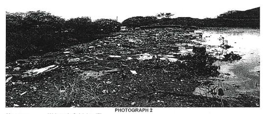
Site name: Location: Date taken: Photographer: Description: Waimanalo Gulch Landfill 94-460 Farrington Highway January 13, 2011 JRuiz Western view of the sedimentation basin overflow spillway area, overtopped with large amount of trash and debris.
