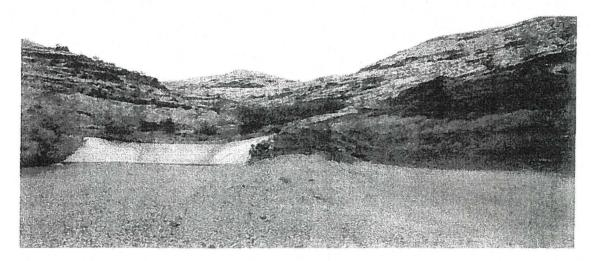
Site Name:Waimanalo Gulch MSWLF and Ash MonofillLocation:92-460 Farrington Highway, Kapolei, Hawaii 96707Date Taken:August 2, 2006Photographer:JRuizDescription:Wide view of the stormwater channel located at the topside of MSWCell 11 to divert run on water during inclement weather.
