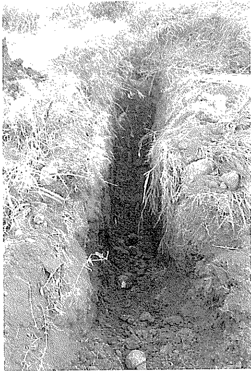
Figure 16. Overview of T5 in Parcel 64, View to Northwest
