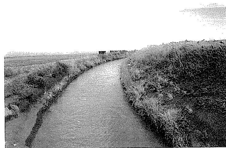
Figure 6. Top: Overview of the New Hamakua Ditch, View to West. Bottom: New Hamakua Ditch, View to North.
