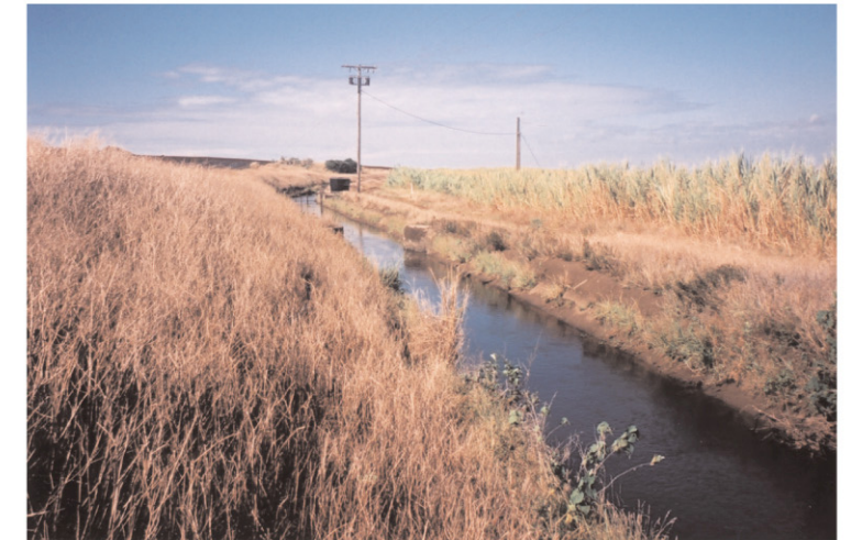
2. The New Hamakua Ditch bounds the property on the northwest and southwest edges.
