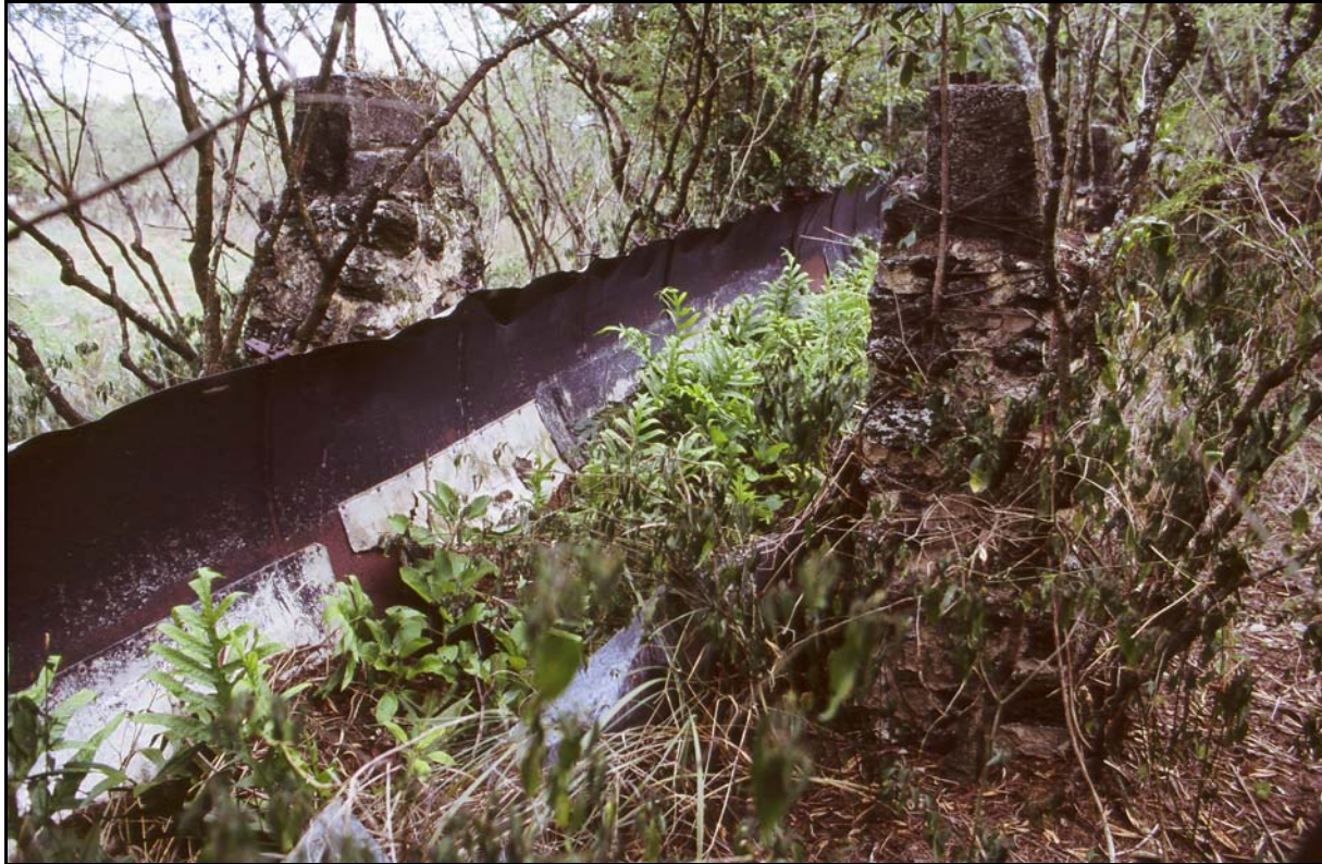
Figure 14. Representative view of elevated plantation-era metal flume. View to the west.
