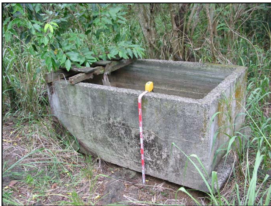
Figure 5. Modern concrete water trough located within the project area.
