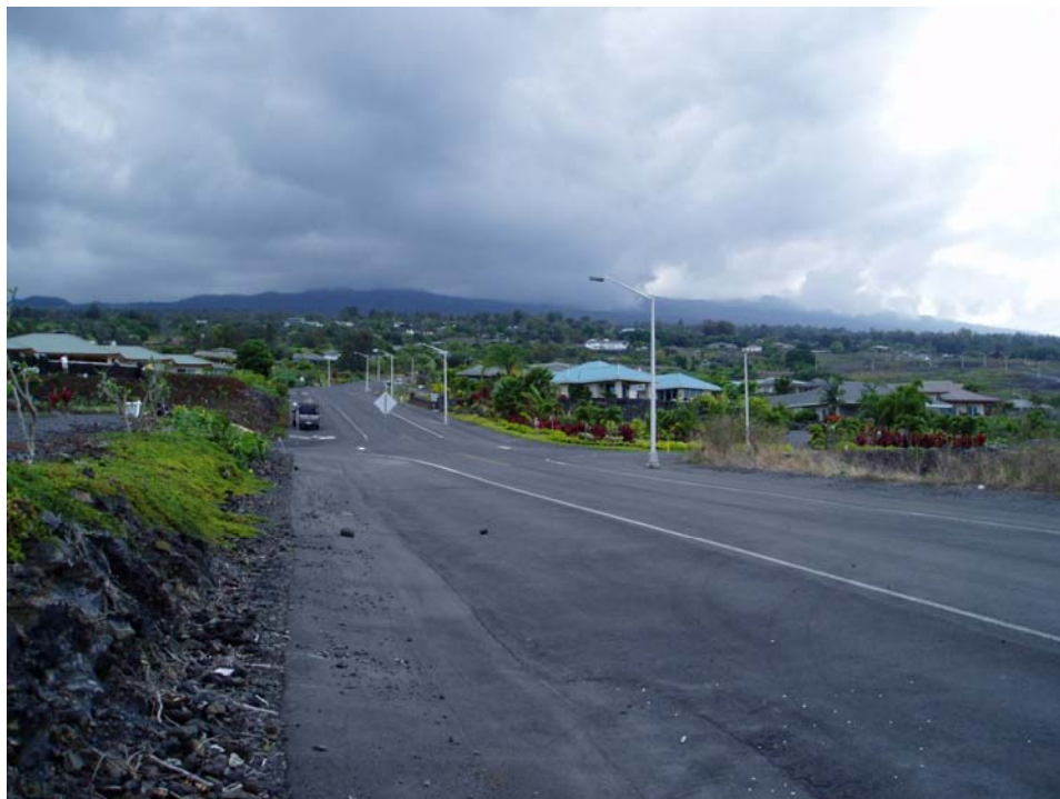
Figure 4-25 View of the Existing Kona Hills Estates Subdivision Adjacent to and East of the Primary Project Area
