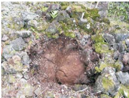
TU-4 base of excavation, view to south
