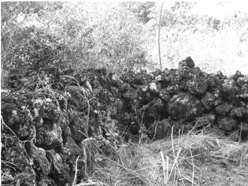
Figure 27. SIHP Site 24415, view to southeast of the enclosure's interior northeast corner.
