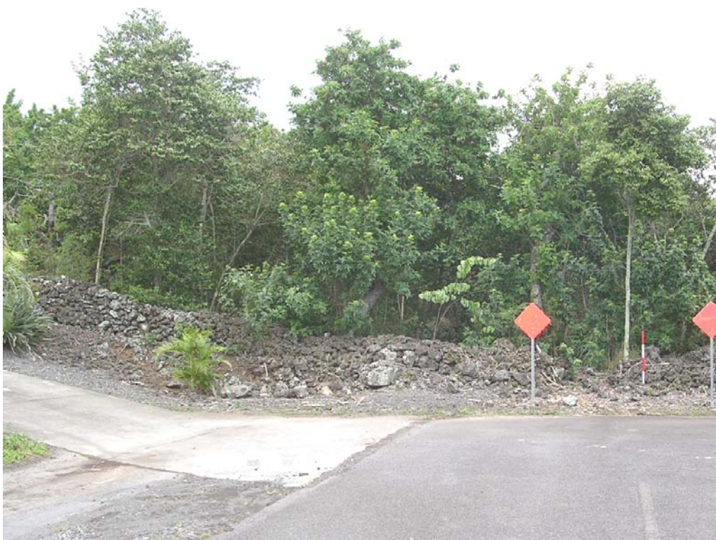
Figure 17. SIHP Site 23834 at the termination of Holoholo Street, expanded view to south (note restacked portion of the wall at the left of the photograph).
