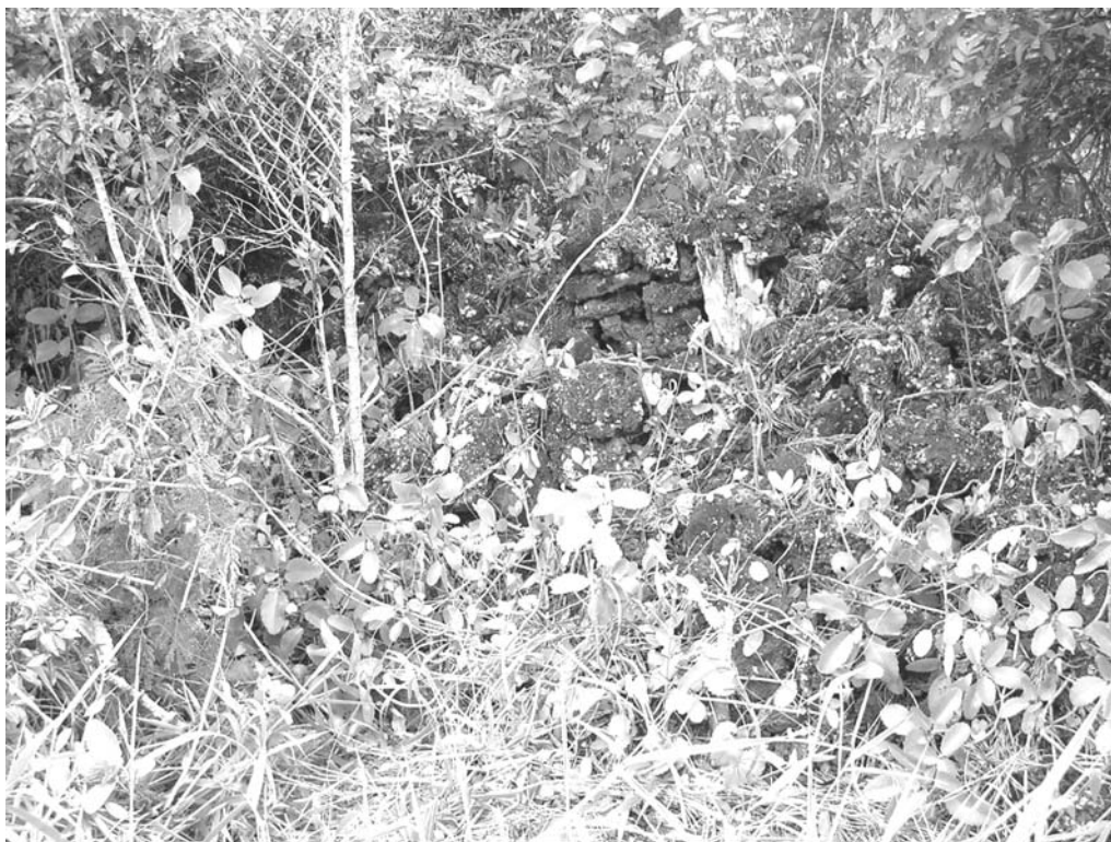
Figure 46. SIHP Site 16125 eastern boundary wall, view to the east.
