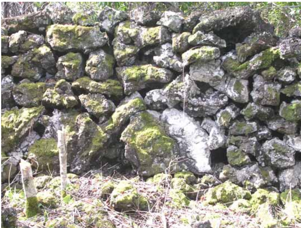
Figure 19. SIHP Site 25527, close-up of wall's northern edge, view to south.
