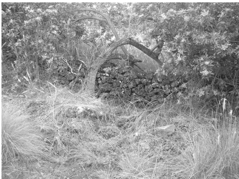
Figure 41. SIHP Site 16106, southern boundary wall, view to the southeast.
