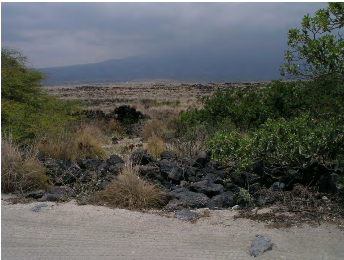
Figure 29. SIHP Site 1911 collapsed western wall of enclosure in foreground and stacked eastern wall in background. The heavily utilized road is immediately adjacent to the site.
