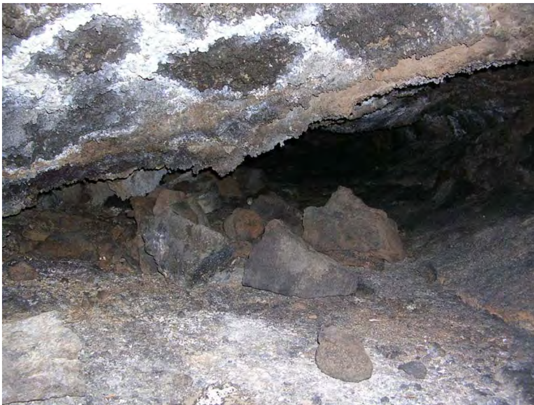
Figure 41. Figure 36. SIHP Site 18027 Feature M, view to the north.
