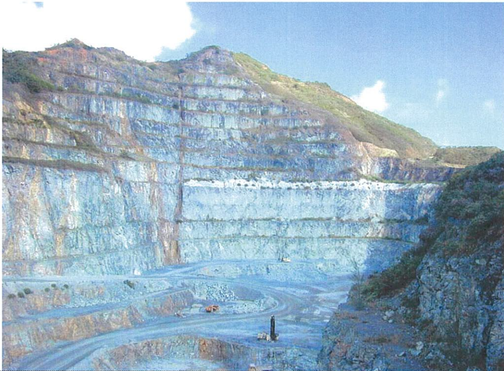
Figure 13. Ameron International quarry pit at Kapa'a. Only minimal vegetation grows in the pit area, proposed as landfill site.
