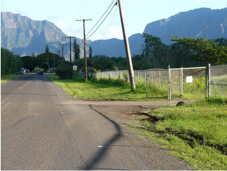
Tropic Land entrance facing the Naval Reservation at the end of Lualualei Naval Road
