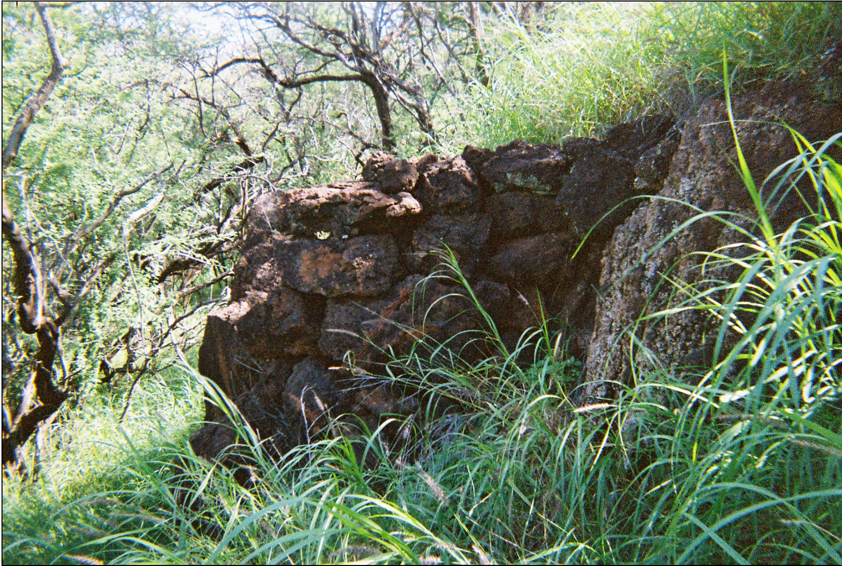
Figure 22: Photographic of Site -6241 Wall Profile. View to East.
