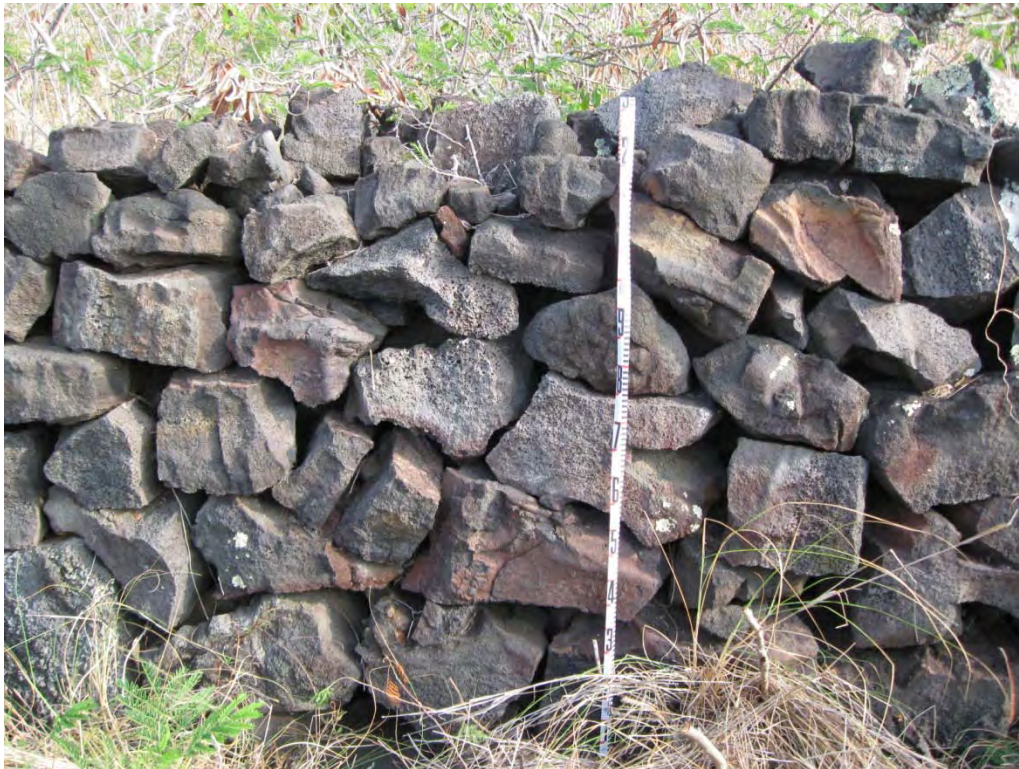
Figure 10. Site 5011 Wall, view to south
