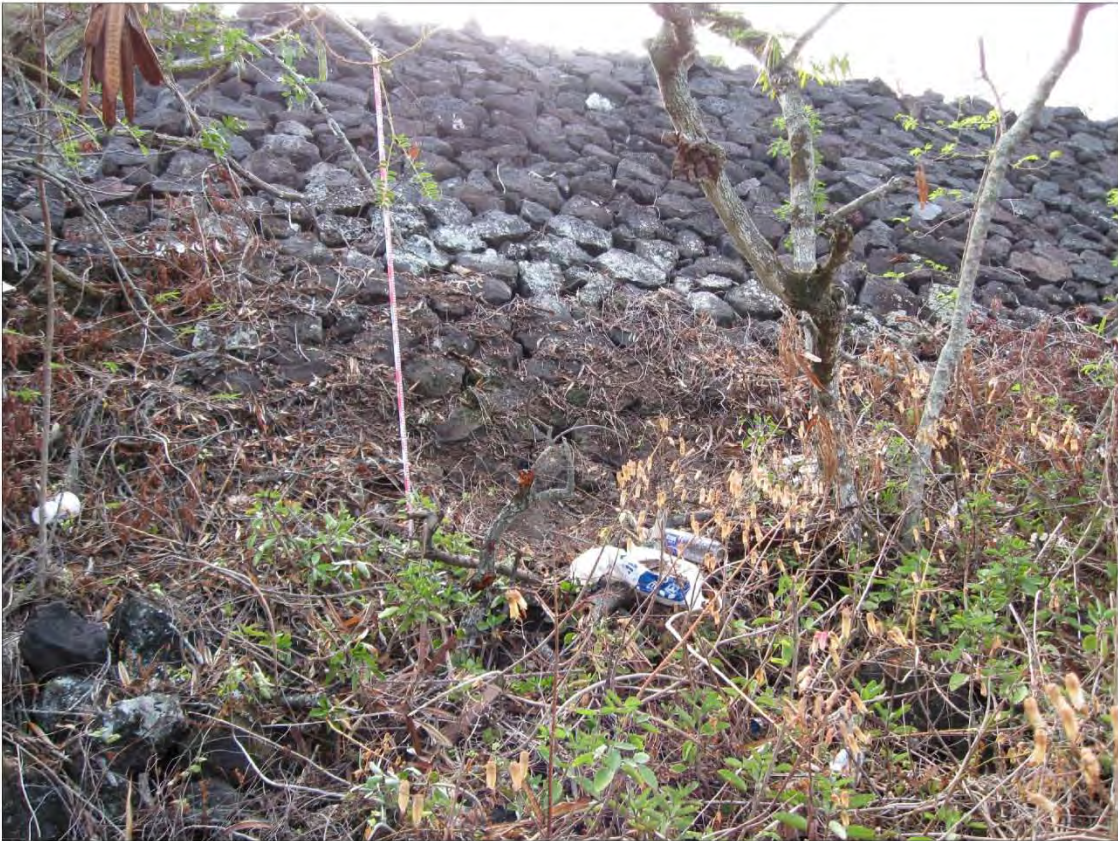
Figure 15. Site 13426 Retaining Wall along road, view to east
